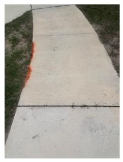
**Action Item Description**Limestone trail: Damaged concrete at sidewalk edge.
